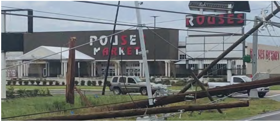
Figure 3. Shoppers buying essential supplies one week after landfall, while the local utility still had no power. Storm structure damage and debris can be seen on the right. The photo was taken by a PowerSecure service technician. Click here to watch a video about PowerSecure’s work with Rouses Market.
